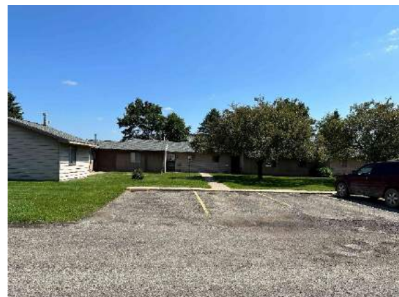
Single-story senior garden apartments in Laingsburg (Looking Glass Terrace)
