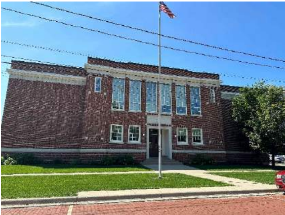
Two-story adaptive reuse apartments in Owosso (Lincoln House)
