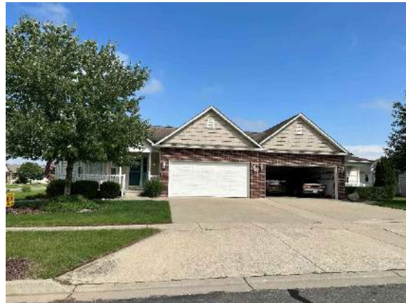
A newer single-story attached home in northeast Owosso
